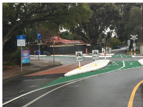
East Ave, Canterbury Terrace and Cromer Parade Intersection
