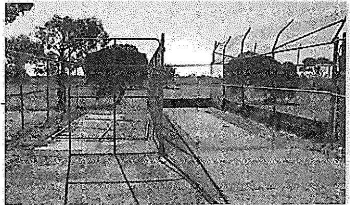
Infill previous safety and maintenance hazard area with compacted granitic sand and 25mm pile synthetic grass.
