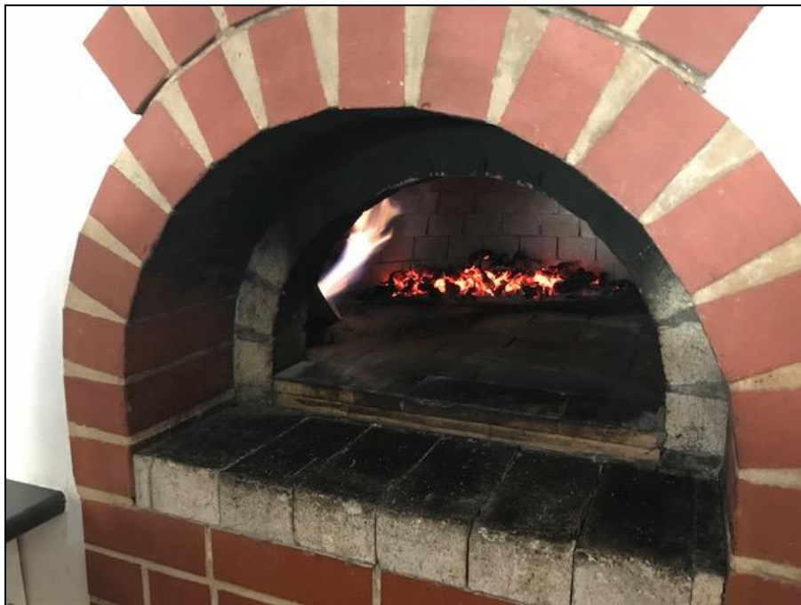
Photo 1: Oven in operation showing embers of wood oven, and gas flame to the left
