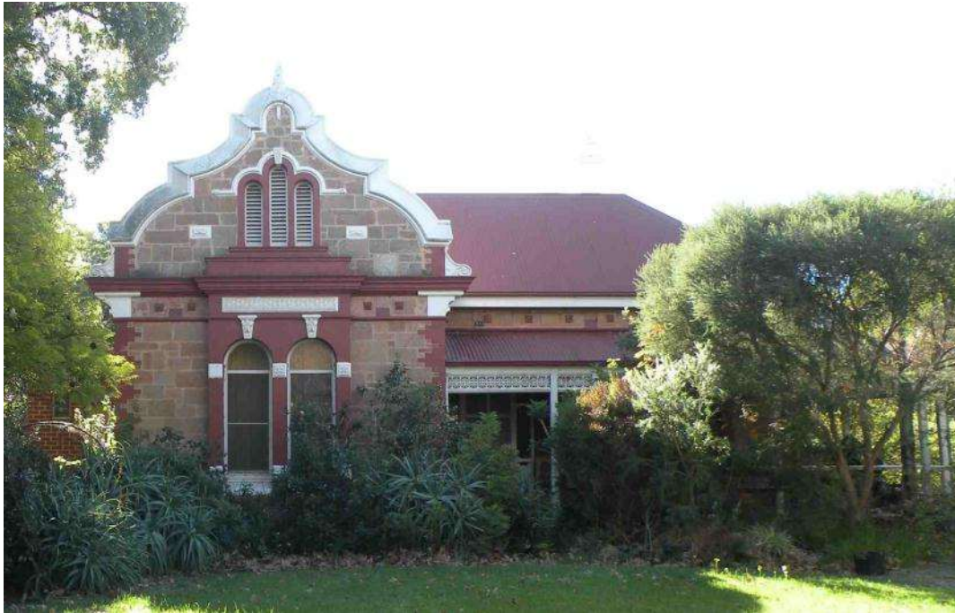
52 Eton Street from south
