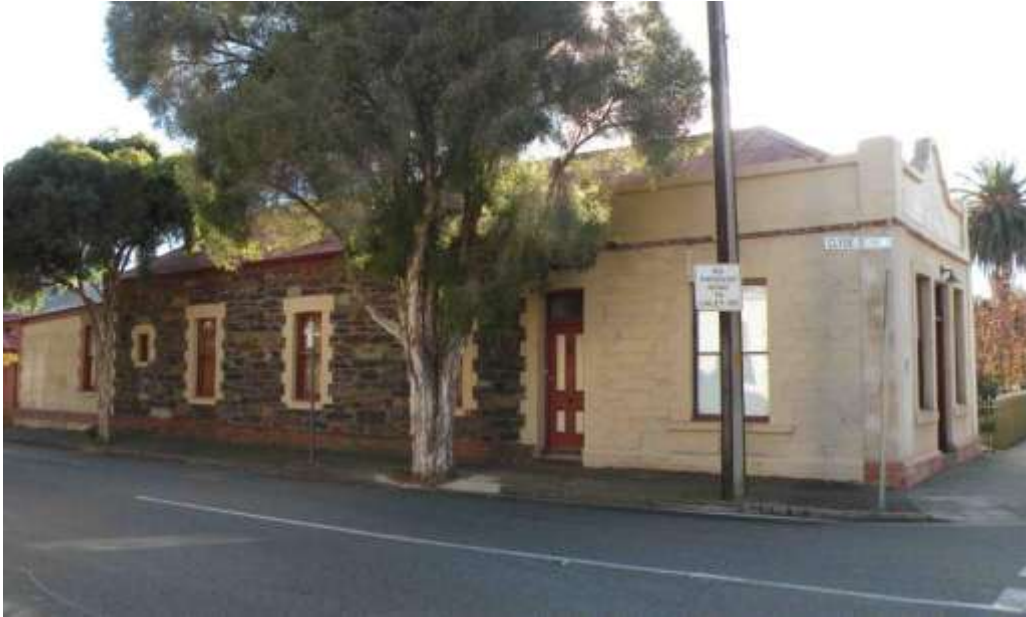
26 Porter Street from south-east
