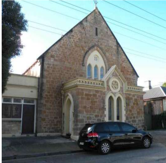
152 Young Street from south-west
