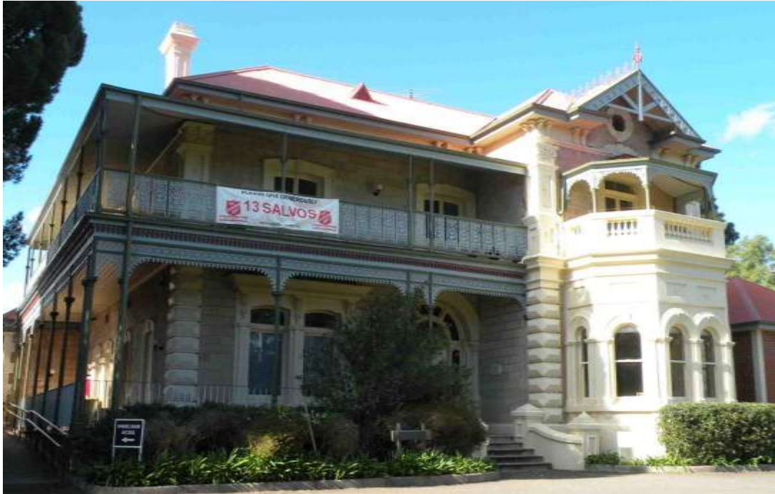
39 Florence Street from west
