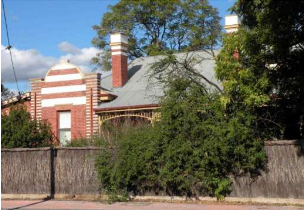
364 Fullarton Road from north
