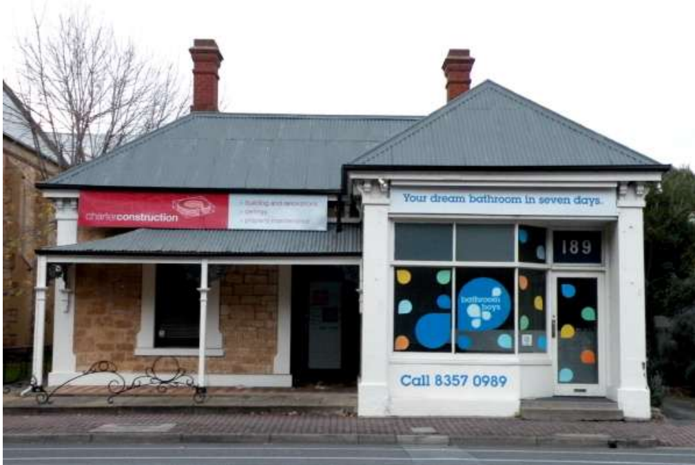
189 Unley Road from west
