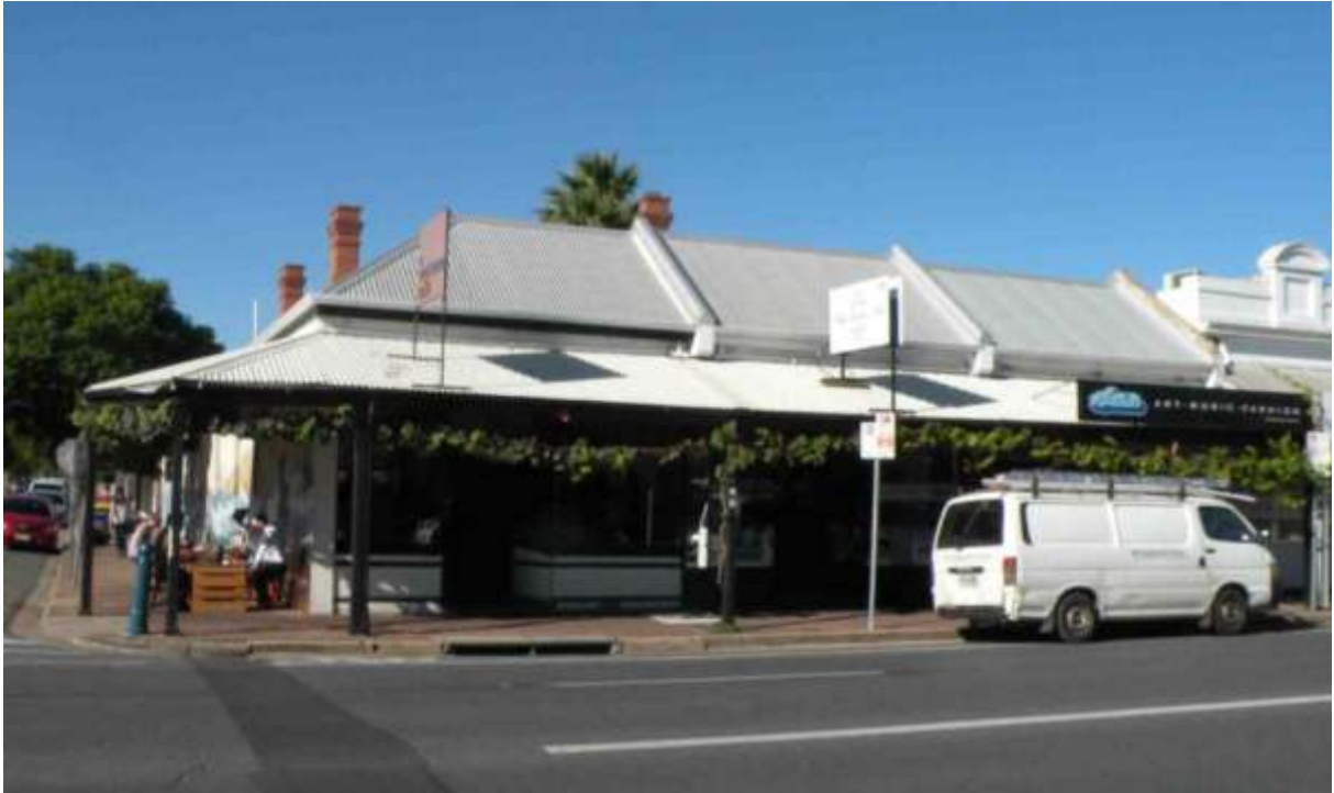
105-109 Unley Road from west
