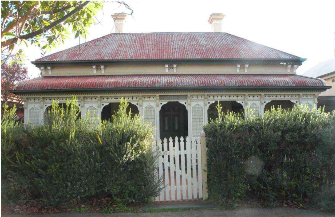
28 Salisbury Street from east
