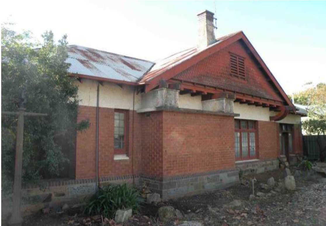
204 Cross Road from south-west
