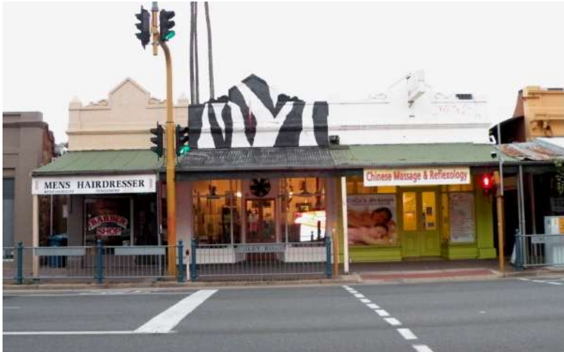
137-141 Unley Road from west
