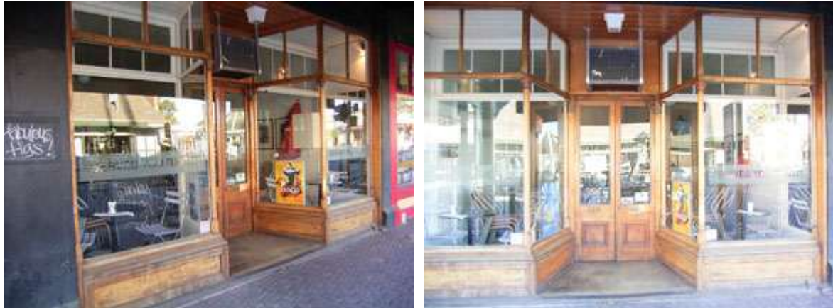
Views of shopfront to number 139 in 2005
