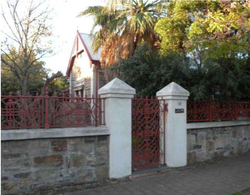
10 Eurilpa Avenue from south
