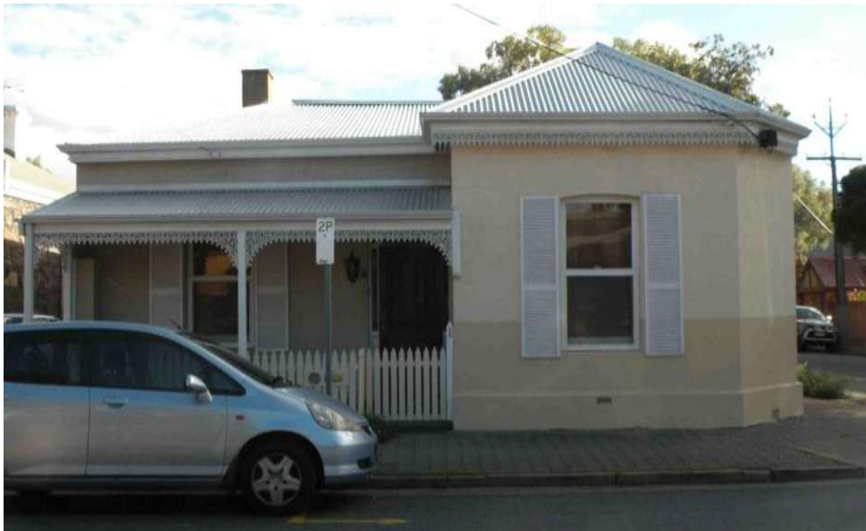
28 Porter Street from east
