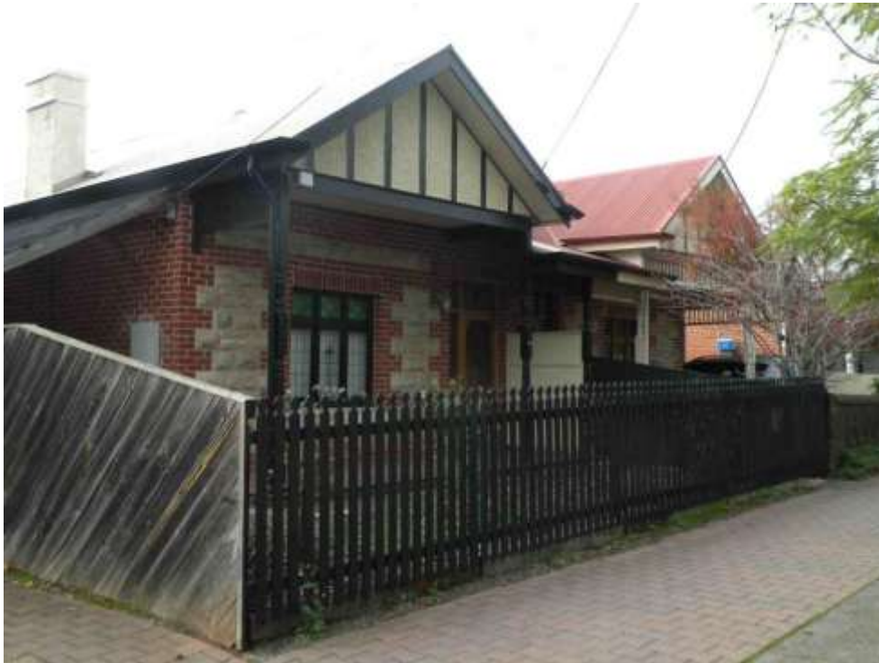
314-316 Young Street from south-west
