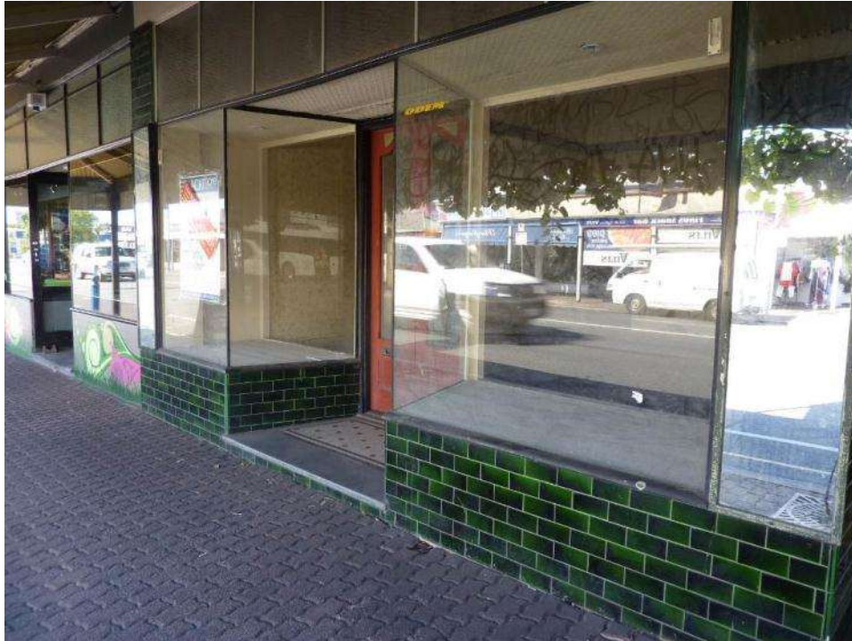
Intact shopfronts to 105 and 107 Unley Road
