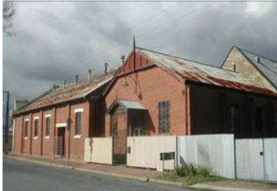
Hall facing Townsend Street
