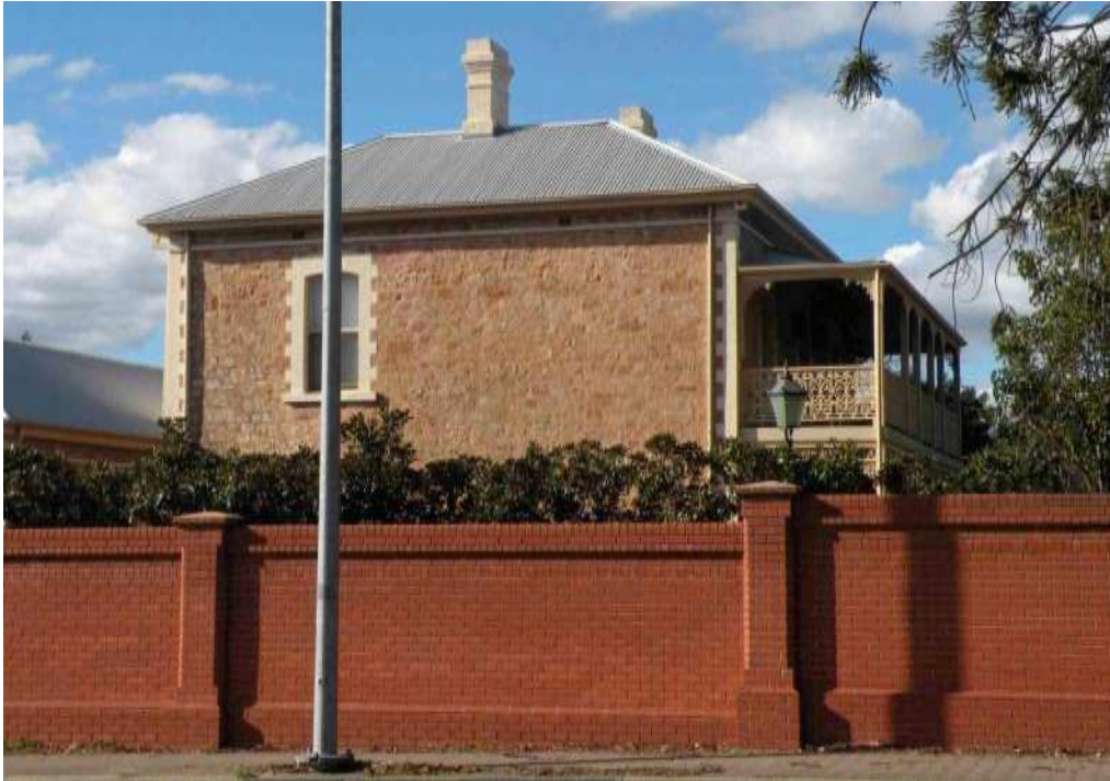
158 Cross Road from west
